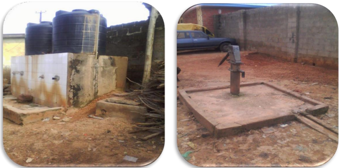
Plate I: Motorised (Cheniyen Ward) and Non-Motorised (Masaga A Ward) Community Water Boreholes
