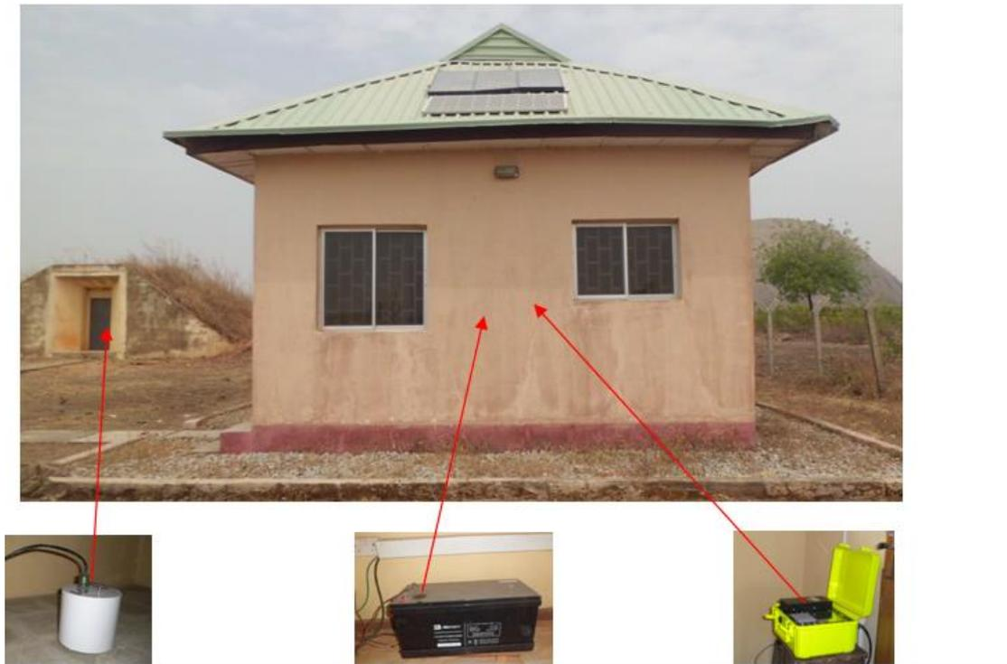
PLATE IV: Kaduna Seismological Station (KAD). (The seismometer [left] is installed in a vault beside the building and the data acquisition system [right] is placed inside the building. The solar panel at the top of the roof is connected to a battery [middle] which supplies power to the seismic equipment. In the background behind the building is an outcrop of quartz porphyritic granite of the Older Granite Complex).
