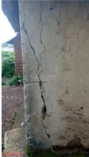
Plate V: Damage to a mud building in Kwoi town
