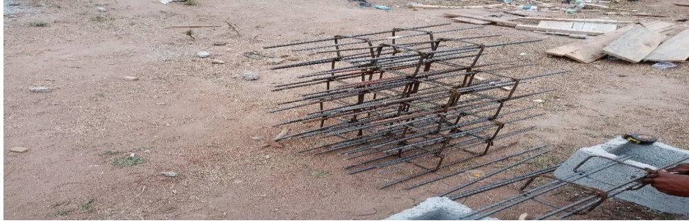
Plate III: Beam reinforcement bars
