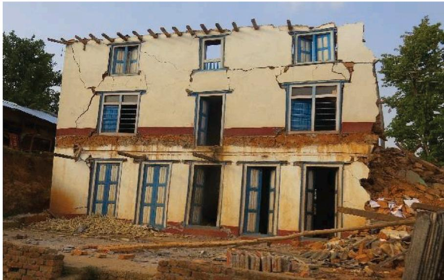
Fig. 1. Observed in-plane failure in piers and spandrels of an URM building [10].
