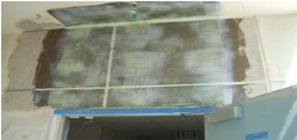
Fig.7: depict the use of advance composite in the healing of concrete spall on wall (Chiewanichakorn & Toranzo, 2011).
