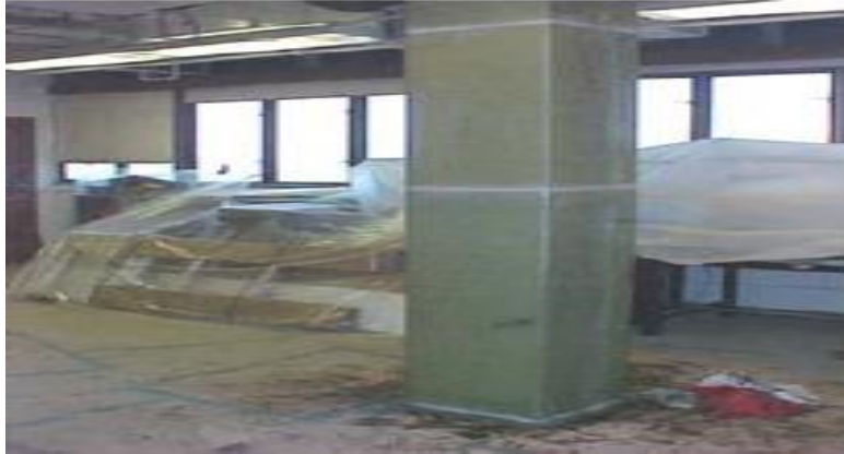
Fig.8: Depict the use of advance composite in the healing of concrete spall on wall (Chiewanichakorn & Toranzo, 2011).
