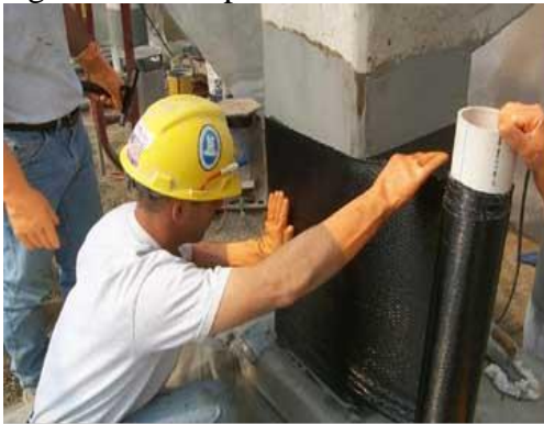
Fig. 7: shows the repair of concrete column with ACM.
