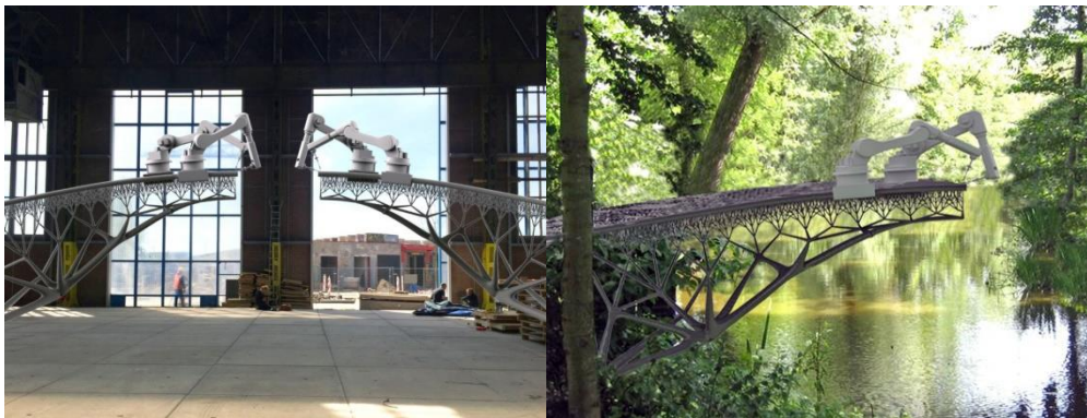
Figure 4: Amsterdam's new 3D-printed steel bridge.
