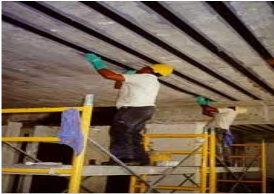
Fig. 6: shows repair of concrete beams with ACM.
