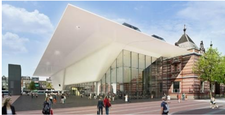
Fig.5: Illustrate the aesthetic possibility of FRP on the city museum façade with free flow of form without column supports.
