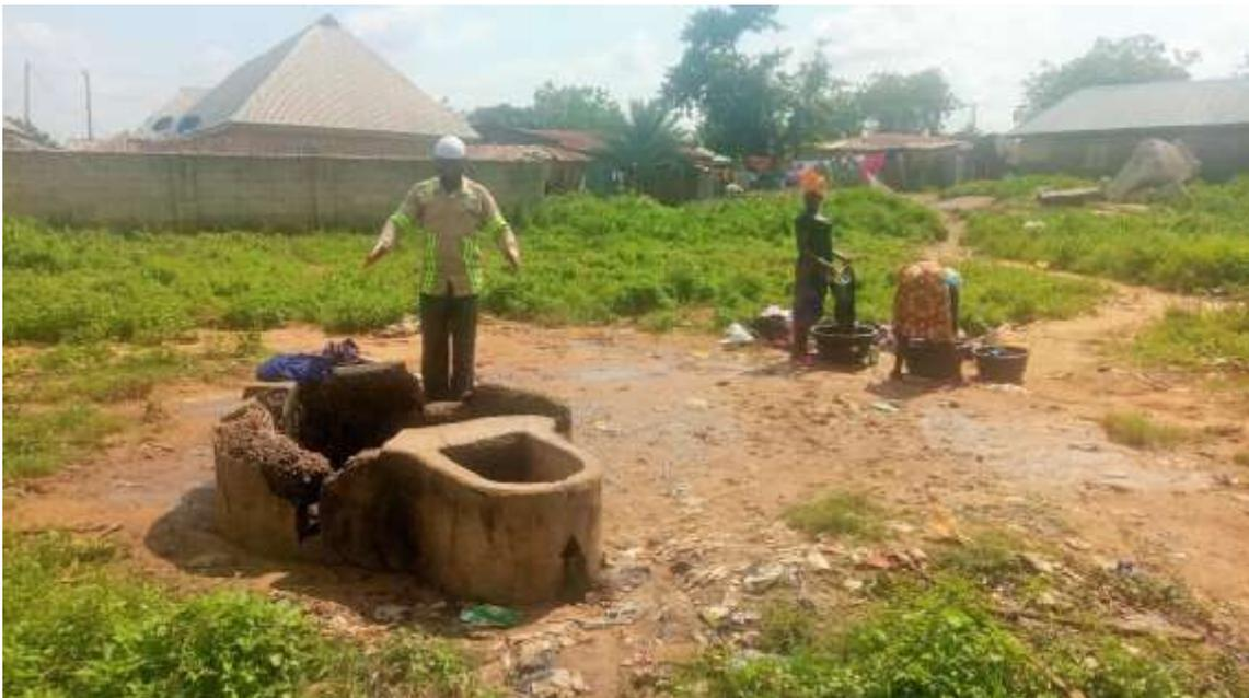
**Plate III. A Typical Poorly Constructed and badly Managed Hand Dug Wells Environment Sampled at Maikunkele, MK1**
