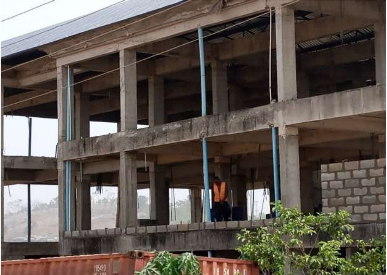
Plate I: A typical structural building under construction with vertical circular pipe passing through a reinforced concrete beam (Abuja – 27/01/2020).
