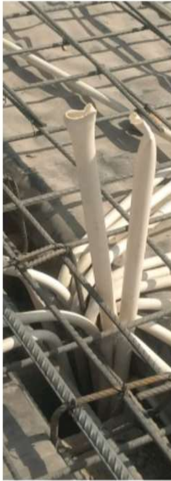
(b) Electrical pipe
