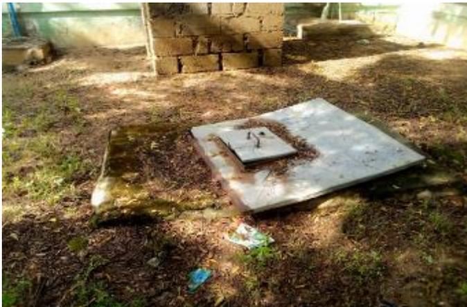
**Plate 9: Showing the damaged sock-away**
