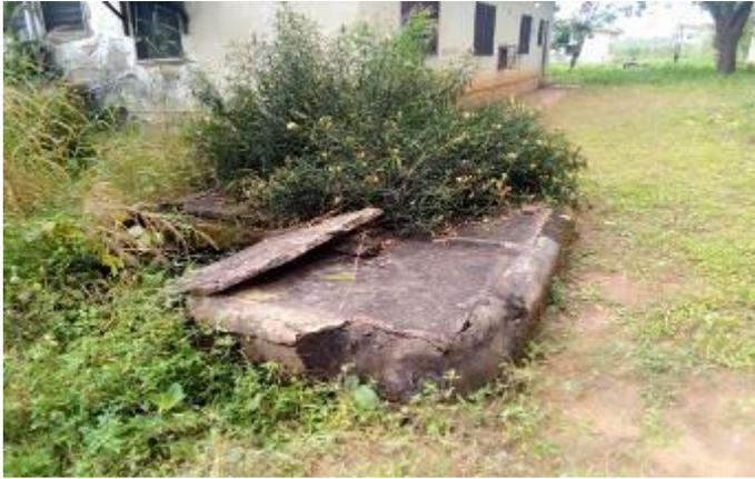
**Plate 8: Showing the damaged sock-away**
