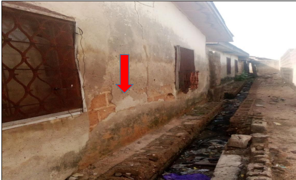
Plate III: Wall condition of rental house in Tunga lowcost Minna
