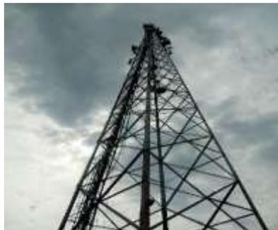
Plate V Tower (For Mounting RF, Microwave Antennas and Terminating Cables)
