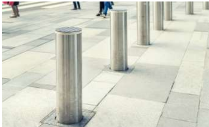
Figure 2.2: Bollard placement as a blockage against vehicle trespassing Source: Zahner, (2017)
