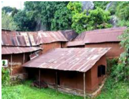
Plate XVIII: Lean to roof used at Oke Idare palace, Akure, Ondo state. Source: (Folarin, 2014)
