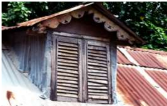
Plate IXX: Dormer roof with carved wooden windows used at Oke Idare palace Source: (Folarin, 2014)
