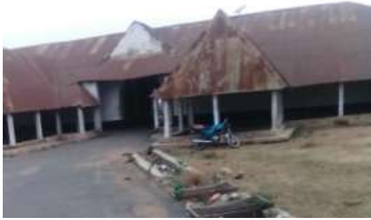
Plate XVII: Gabled roof entrance known as Agaju used in the Alaafin of Oyo Palace. Source: (Author's field work, 2021)
