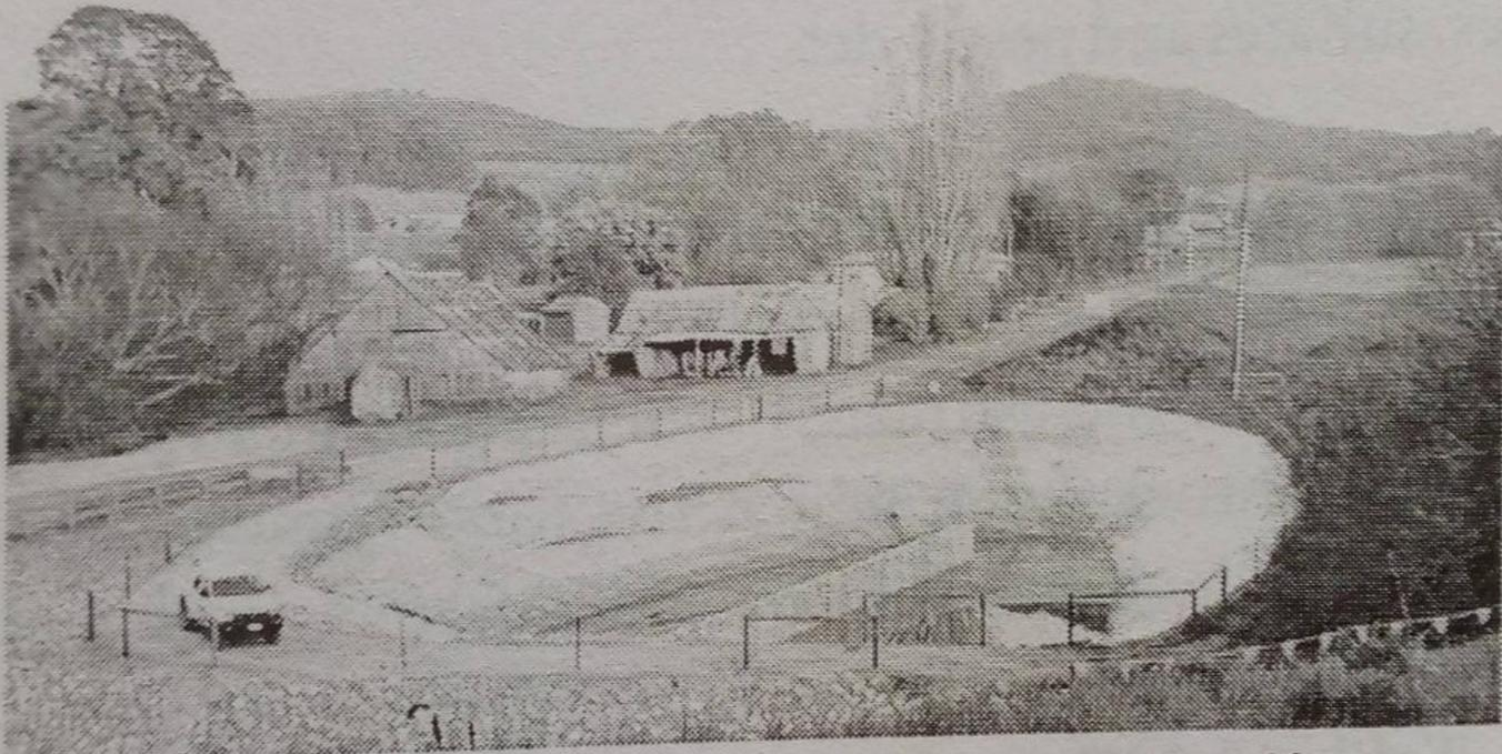
Plate 10.8 Example of artificially made off-stream dam
