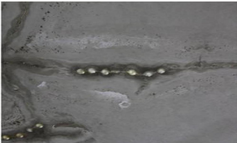
**Figure 1.5: An *in situ* application of bacteria based liquid (Anitha *et al.*, 2018).**
