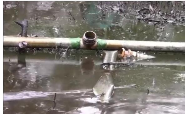
Plate 5: Typical Crude Oil Tapping Point
